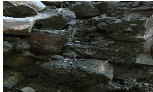
Fig. 8. Fibers helps in bonding with concrete
