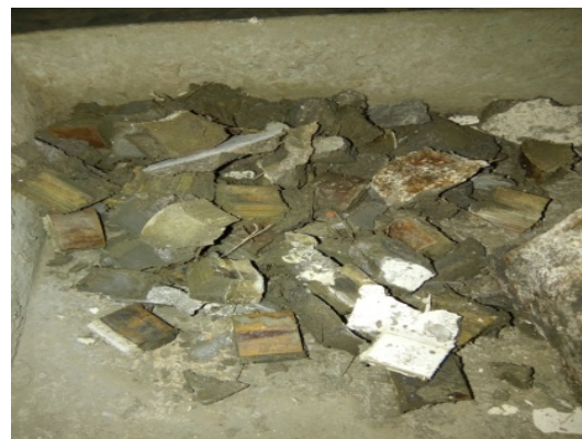
Fig. 9. Failure of mortar without any effect on bamboo aggregates.
